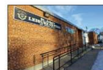
St. John's Leisure Centre 601 Aikins Street R2W 0J9
